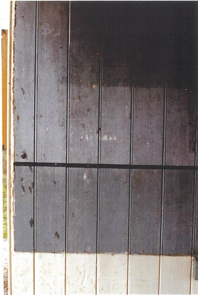
Figure 5.1 Maindample: detail view showing use of Grey/Blue and Light Grey. (A. Ward)
