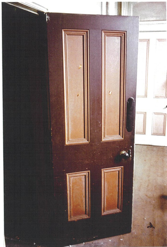
Figure 7.3 Korrumburra: the Kitchen door off the Refreshment Rooms, showing dark leather rails and light leather panels.
