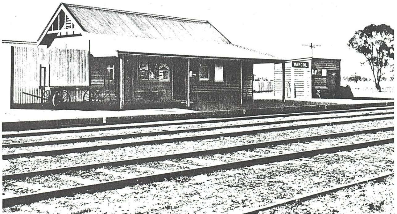
Figure 2.1 Wakool: an example of an unpainted station building. Note the corrugated iron which is also unpainted. (STA 32/2)
